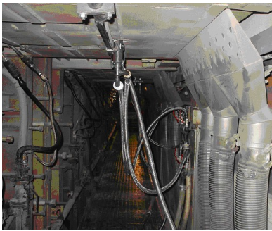
Fig.5 Installation in the port bottom
