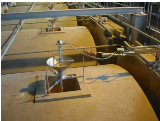
STG Oxygen Sensors: the basis for Lambda Control. Installed in more than 200 furnaces worldwide
